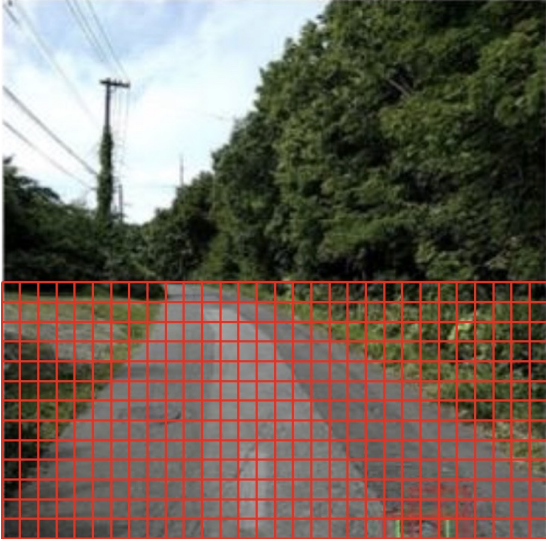
Fig. 5. Cells for road surface damage detection.
